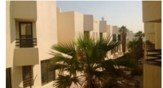
Al Masif Compound (Riyadh) Leasable area 6,838 sqm 26 villas. 0% leased
