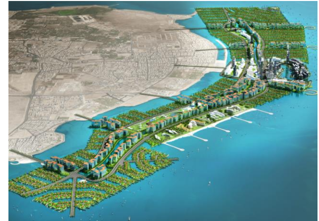
Juman Project - Dammam
